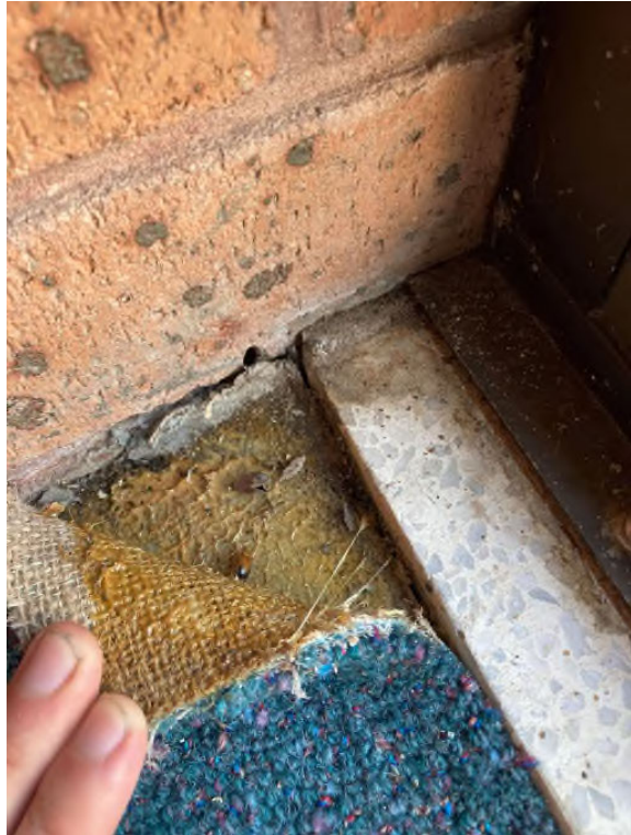
Representative photograph of the flooring beneath the carpet within Meeting Room 2, at the time of the inspection
