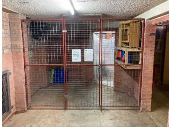
Representative photograph of the padlocked room within the basement, at the time of the inspection
