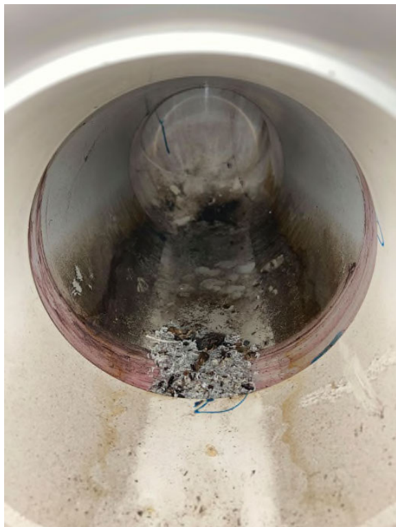
Representative photograph of one of the L-shaped pipes within the southern room of the basement, at the time of the inspection
