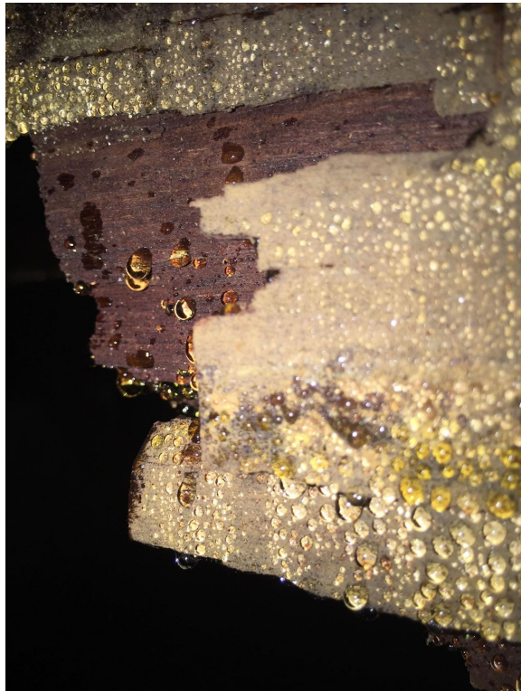
Representative photograph of one (of many) of the floor timber joists
