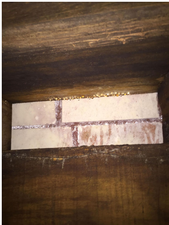
Representative photograph of the northern brick wall within the subfloor
