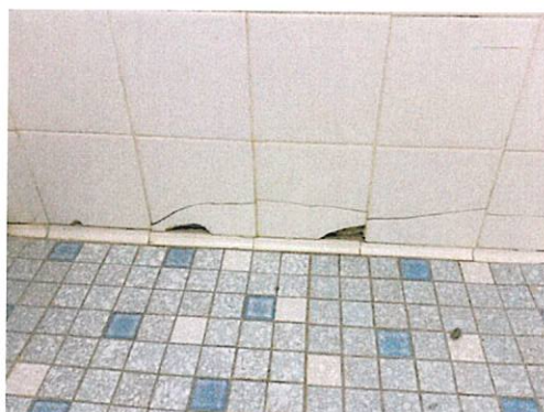
Wall Finishes - Ceramic Tiles
