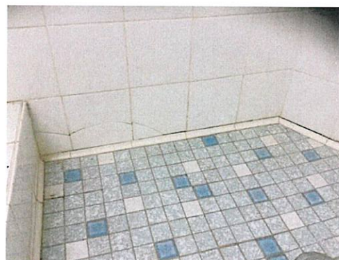
Wall Finishes - Ceramic Tiles
