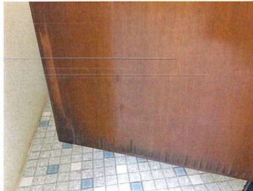
Interior Doors - Polyurethane Finish
