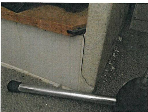
Interior Walls - Toilet Partitions
