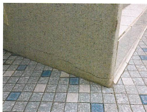
Interior Walls - Toilet Partitions
