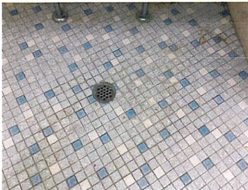
Floor Finishes - Ceramic Tiles
