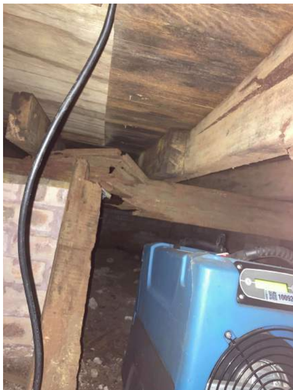
Representative photograph of one of the timber bearers within the basketball court subfloor, at the time of the inspection
