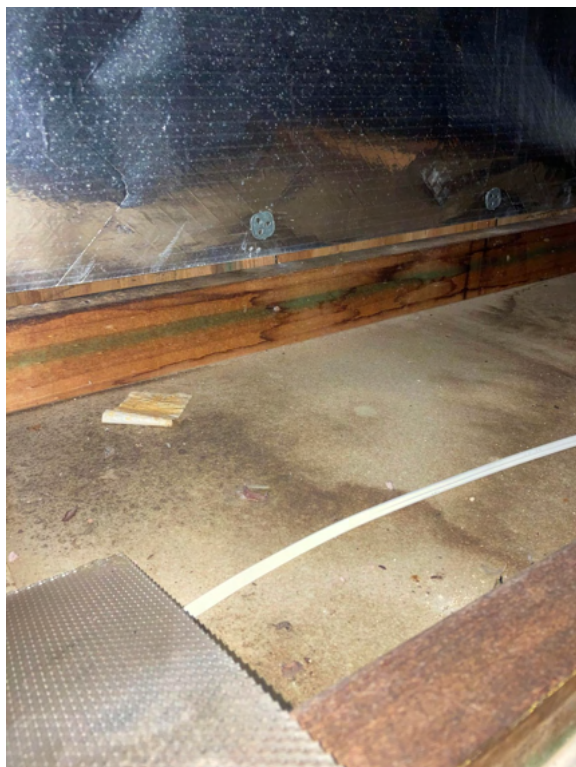
Representative photograph of the horizontal ceiling cavity surfaces within the structure, at the time of the inspection
